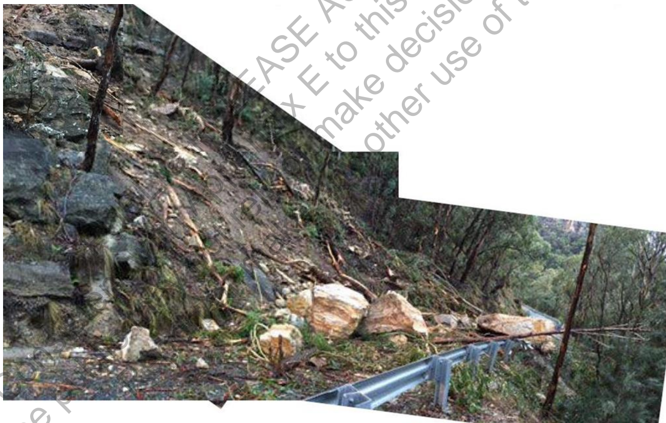
Figure 8: Debris left on road following rock topple within Domain 1 in June 2016.
